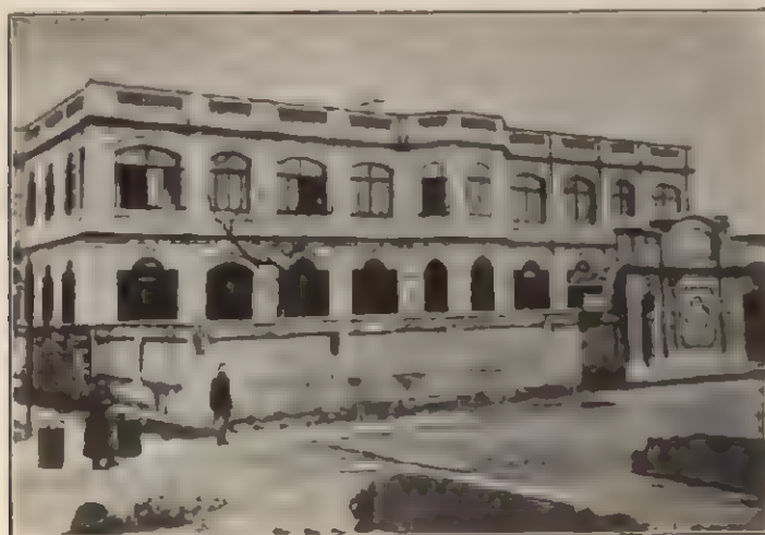
FIG. 325 The Christian Hospital, Shaohsing. Just completed.
