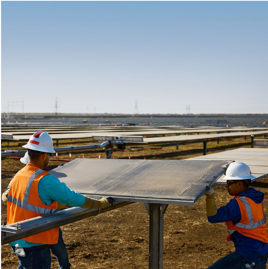
Apple is investing in renewable energy worldwide — including this large-scale solar project in Brown County, Texas — to help address the electricity customers use to charge their Apple devices.
