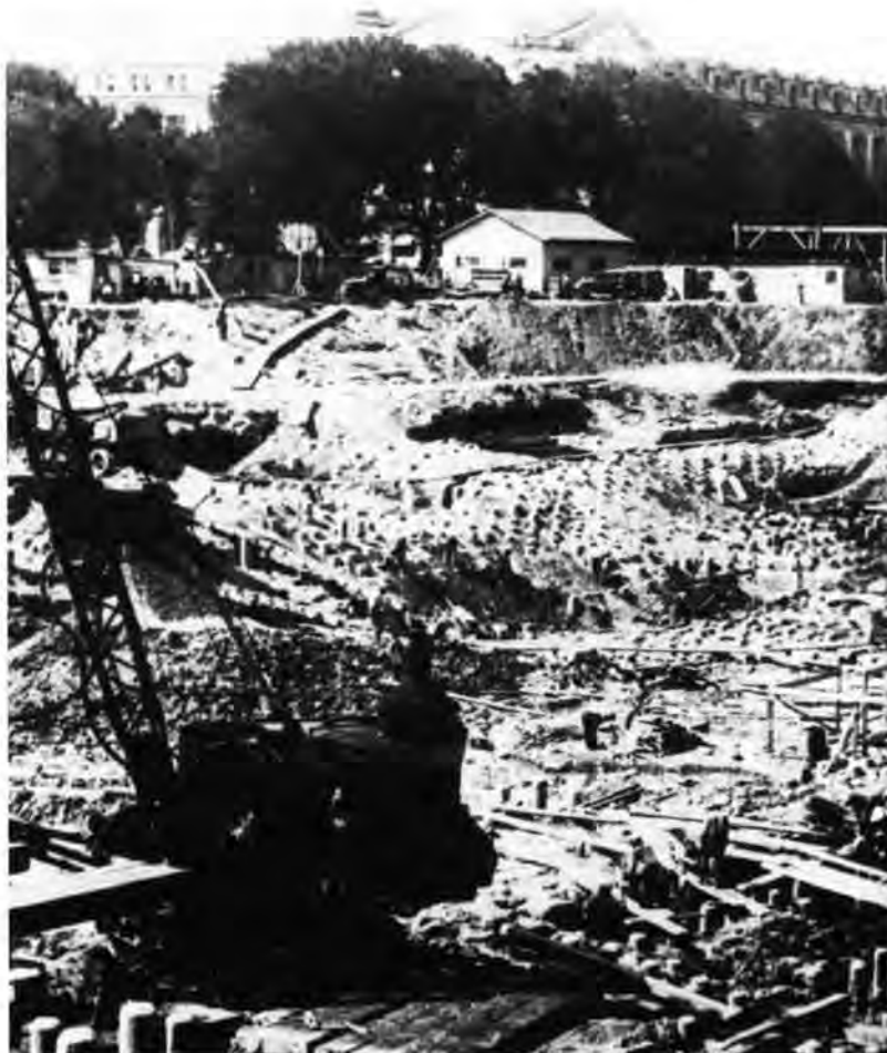
Marshy soil and an underground stream forced the construction crew a bowl to insure a stable building.
