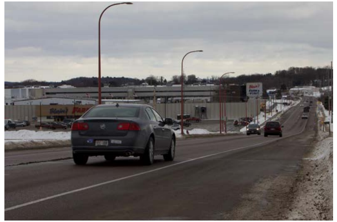
A view of the edge markings on South Boulevard.
