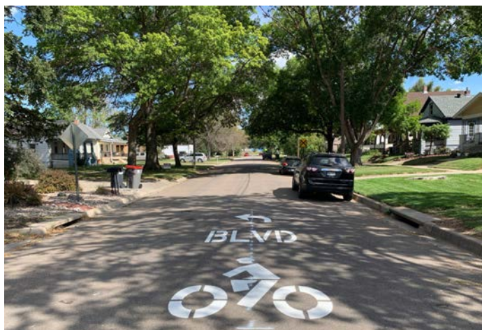
An example of a Bicycle Boulevard (City of Lincoln, NE).
