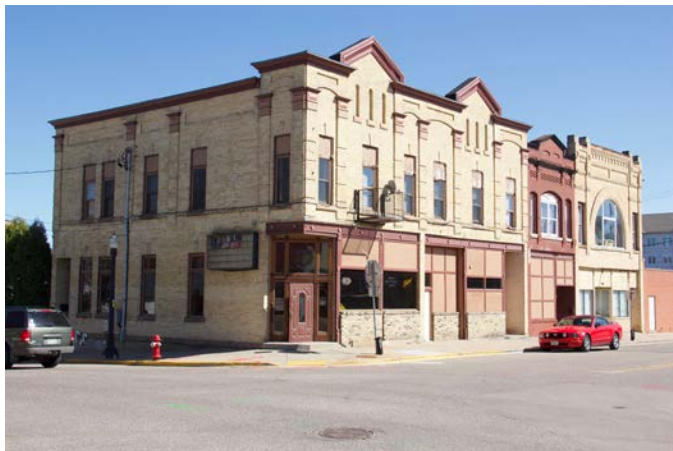
Ash and Water Street, looking Southeast.
