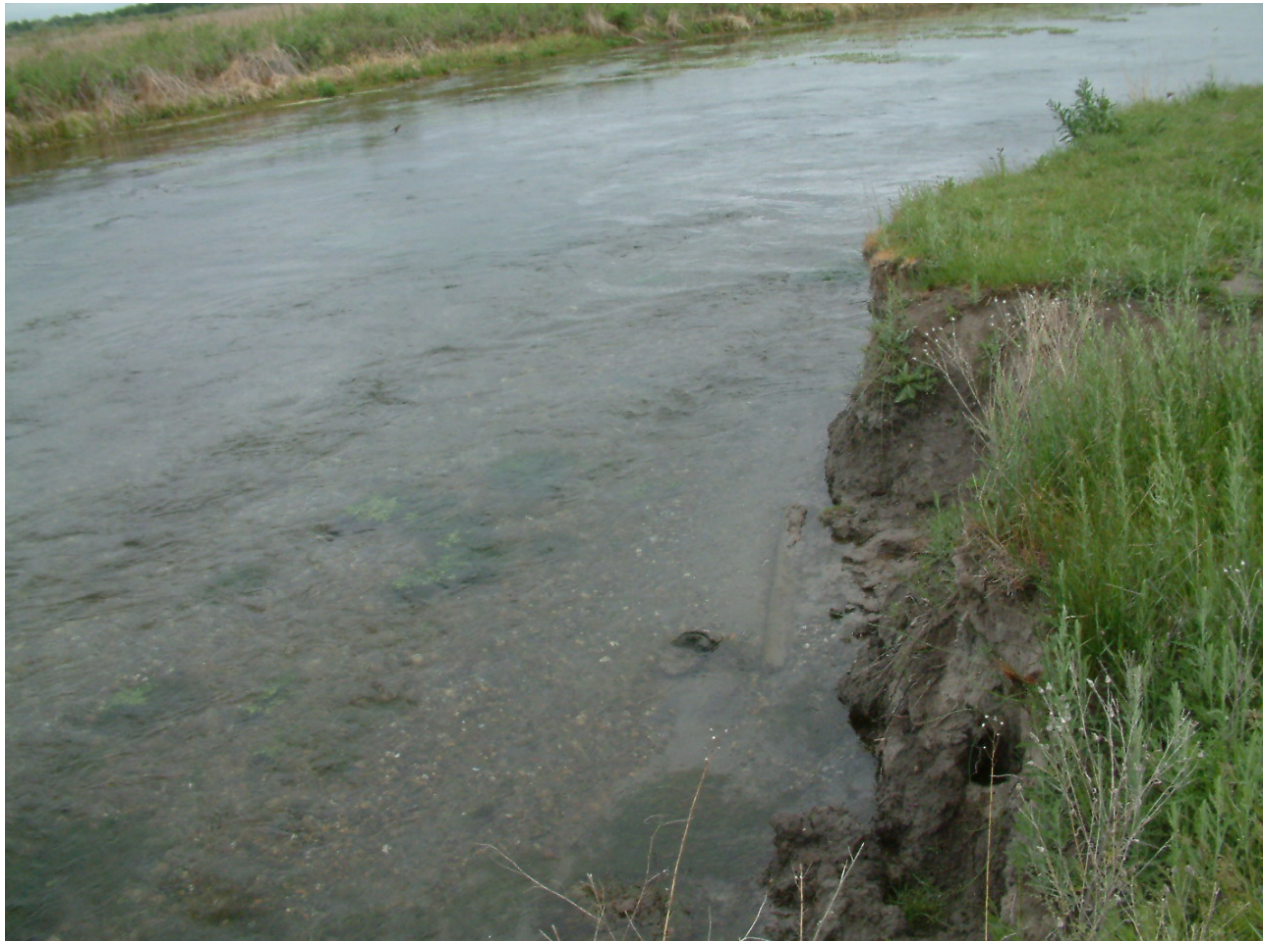
Figure 8. Head-end sloping pre-treatment 2008.
