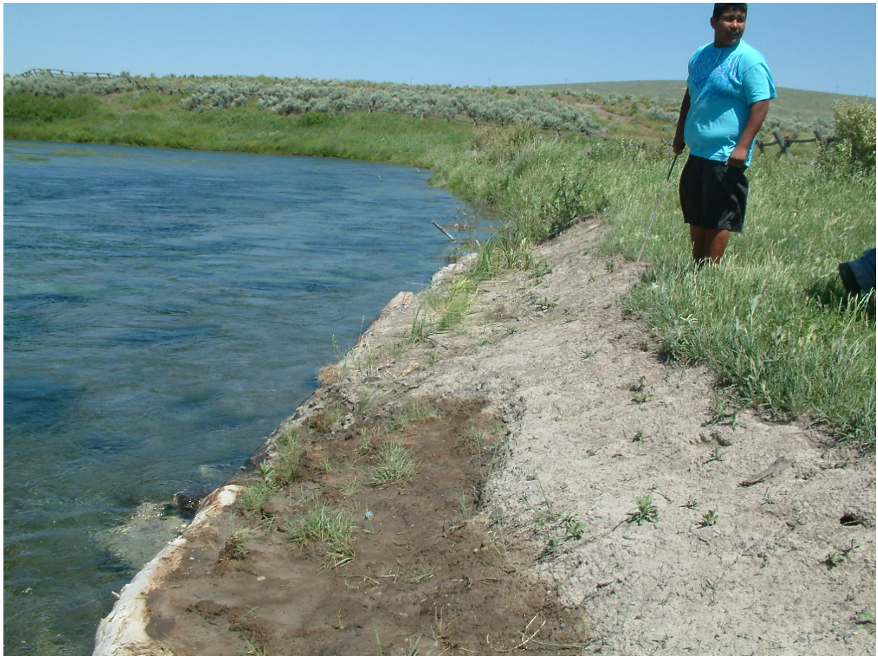
Figure 11. Sloped and planted streambank at Head-end site 2009.
