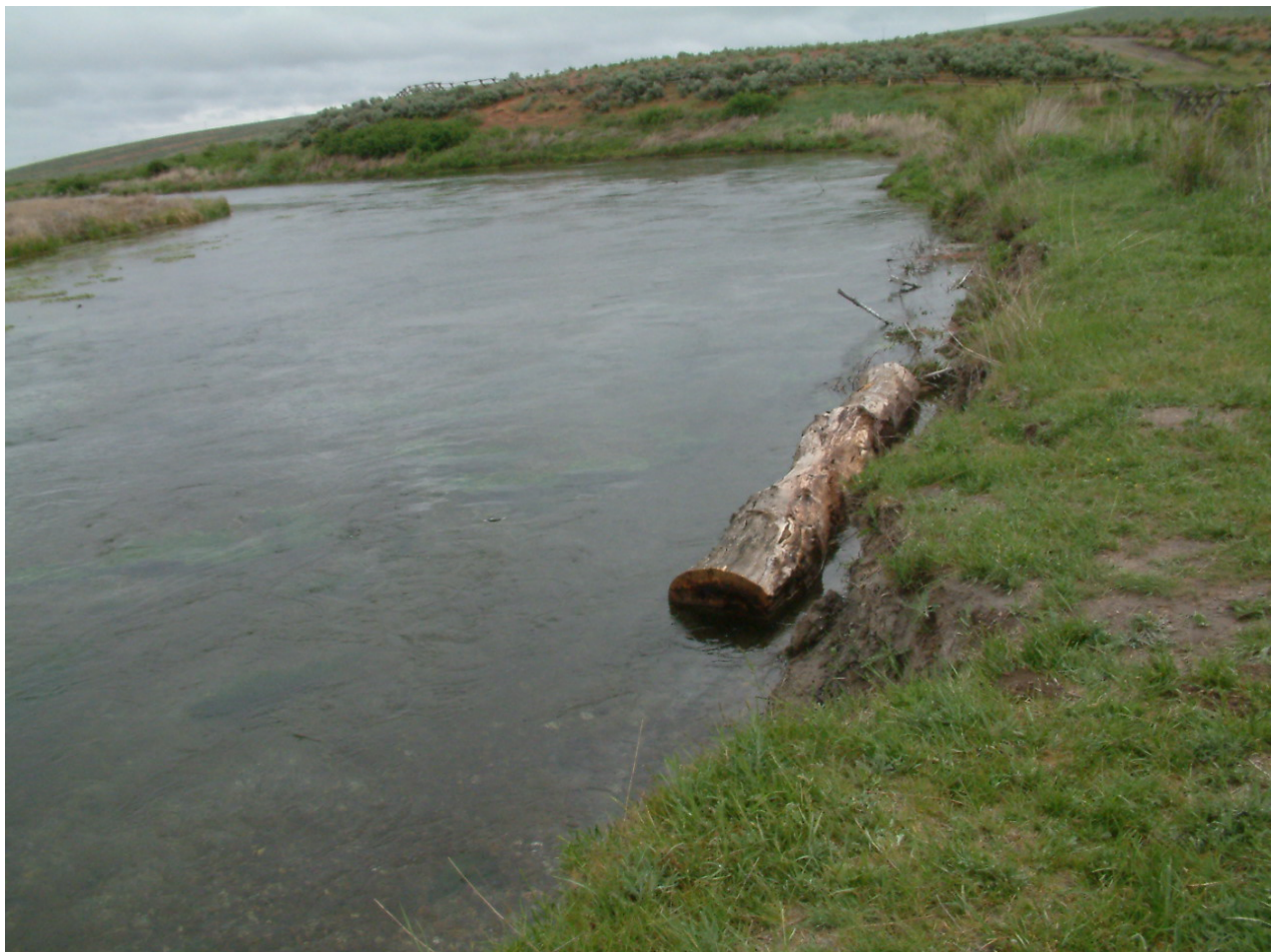
Figure 9. Beginning Phase of stabilization process at Head-end.
