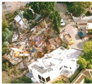
Hillside homes collapsed in the 1994 Northridge Earthquake. PHOTO COURTESY OF CITY OF LOS ANGELES DEPARTMENT OF BUILDING AND SAFETY
