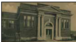
Original Mill Street Façade
