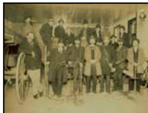
Firefighters in the old Fire Hall
