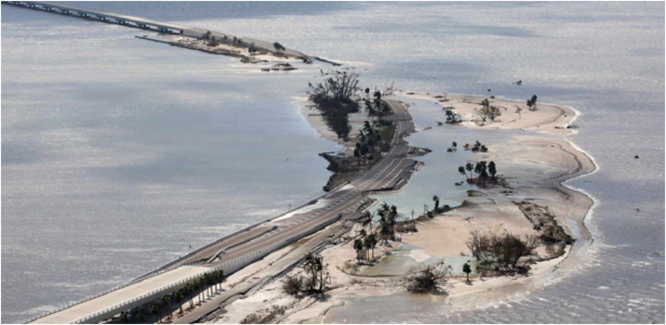
Damage caused by storm surge along the Sanibel Causeway in Florida during Hurricane Ian in September of 2022. Credit: Getty images
