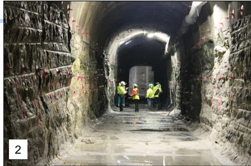
2) Finland – ONKALO: URL for Used Nuclear Fuel – may become part of final UNF Repository
