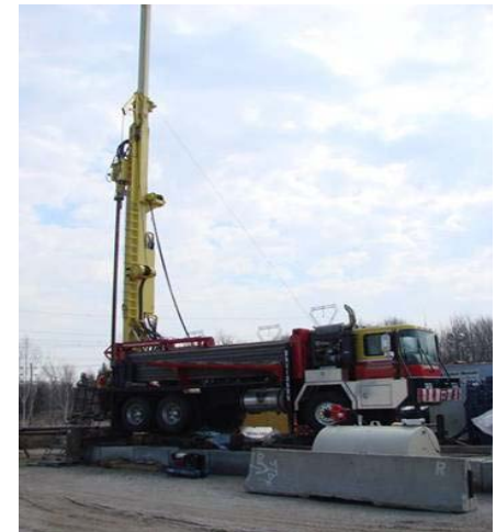
Borehole drilling & testing
