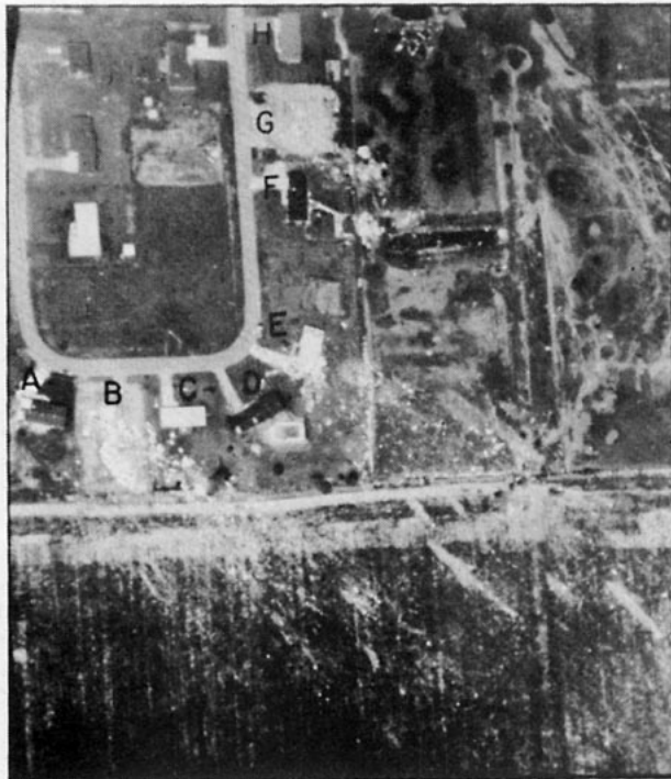
FIG. 20. An aerial view of houses A-H in Fig. 13. Pieces of the roofs were blown into the cornfield, smashing the cornstalks which were about 4 ft tall. Houses B and G were under construction.
