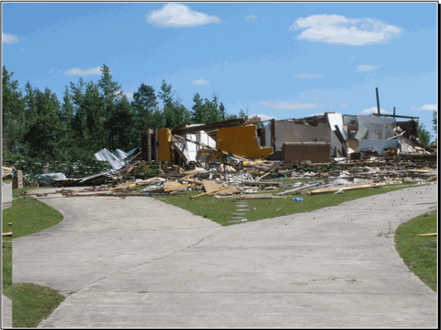
Home destroyed by EF-3 tornado along County Road 32 in northern Choctaw County Alabama on April 27, 2011. Photo by NWS Forecast Office Mobile / Pensacola.
