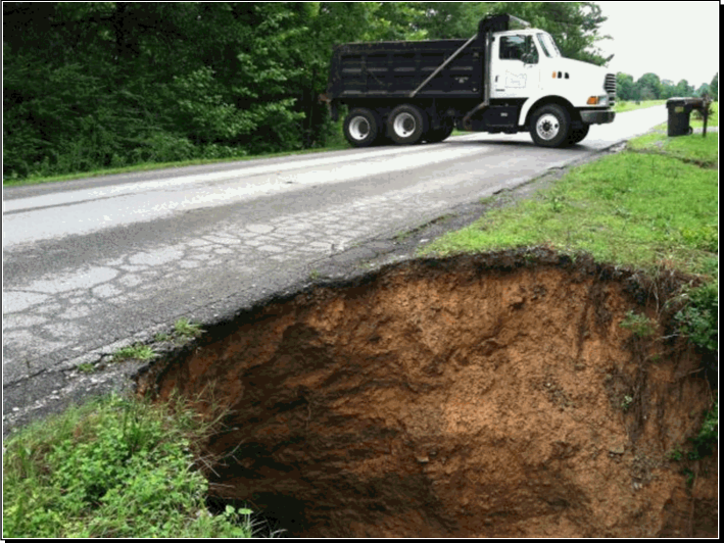
Sinkhole developed along Danville Road from excessive rainfall on July 4th
