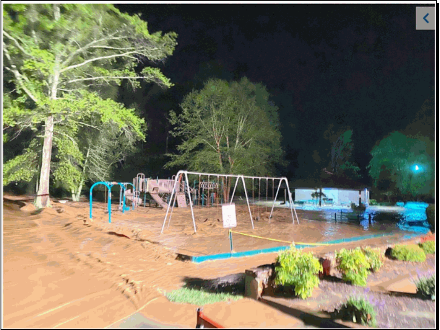
Public Park on AL Hwy 117 in Valley Head inundated by rushing water from flash flooding
