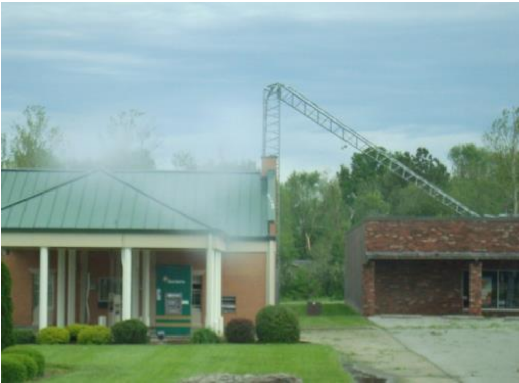
Signs were blown out...
