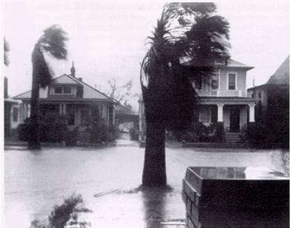
Water and High Winds Damage Galveston Texas, July 27, 1943
