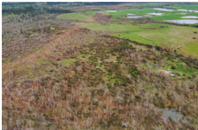
High-wind damage to a rural area in Alabama. Credit: NOAA
