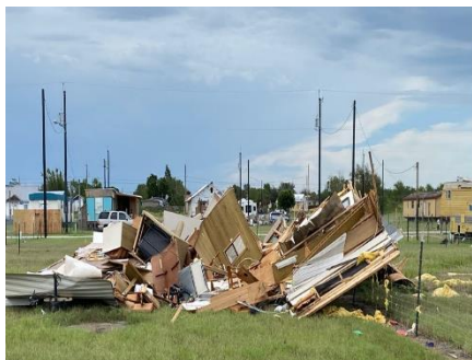
Extensive damage to colonias east of Edinburg, TX, following Hurricane Hanna in July, 2020.
