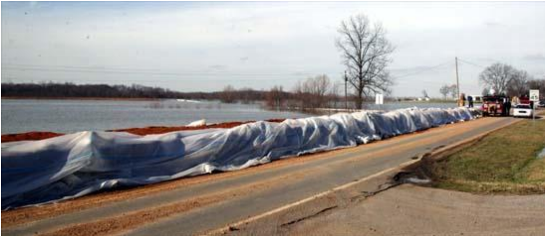
The following photo, courtesy of Beau Dodson, is a view of the makeshift levee constructed on U.S. Highway 60 in Smithland, KY. Photo taken on January 15.
