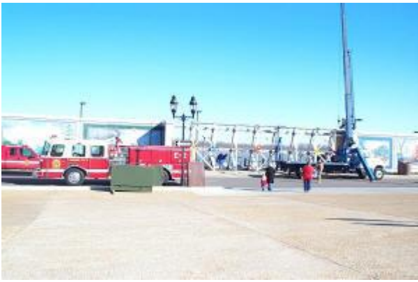
Firefighters and other city workers install a floodgate in downtown Paducah, KY on January 14. This was the first time since the 1997 flood that floodgates were installed in Paducah.
