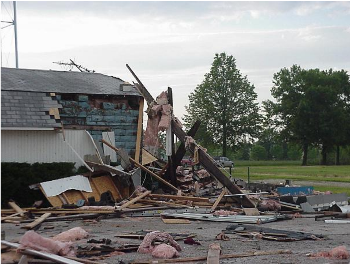
10 bay garage with heavy damage
