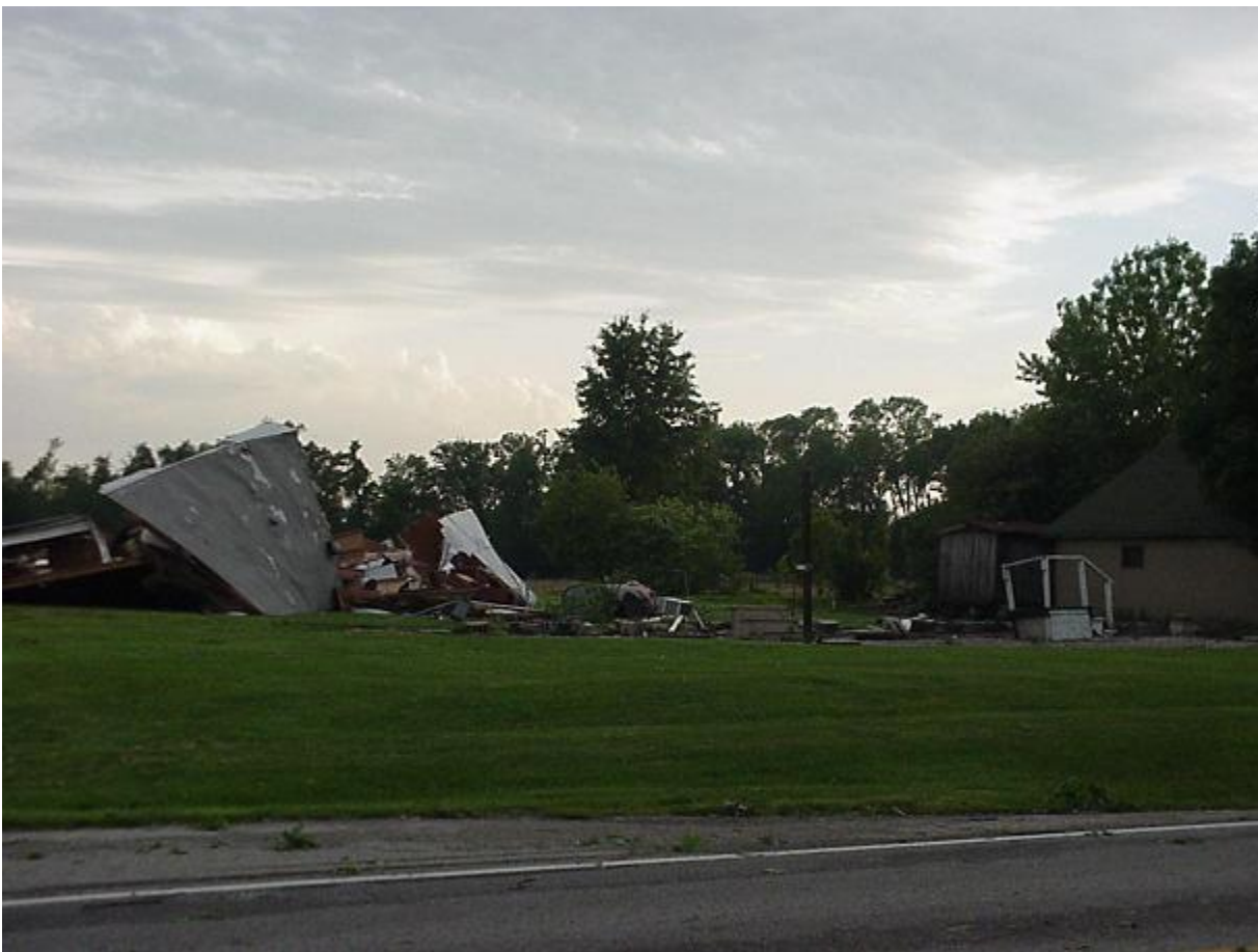
Destroyed mobile home
