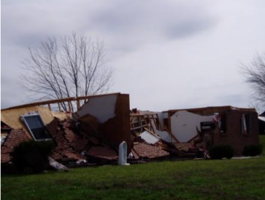
Photo of destroyed brick home near U.S. Highway 61 in Perry County.
