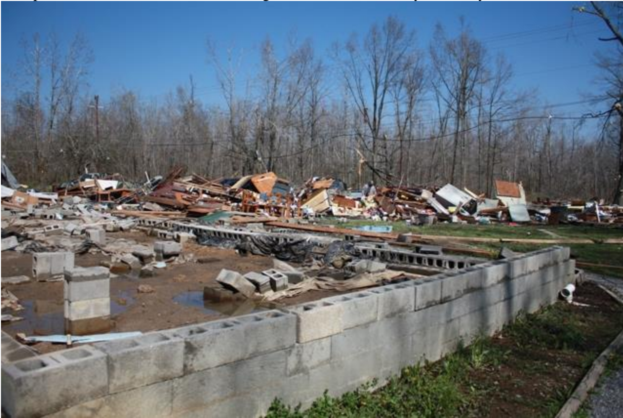
Two photos of home leveled near Mannington, in Christian County Kentucky
