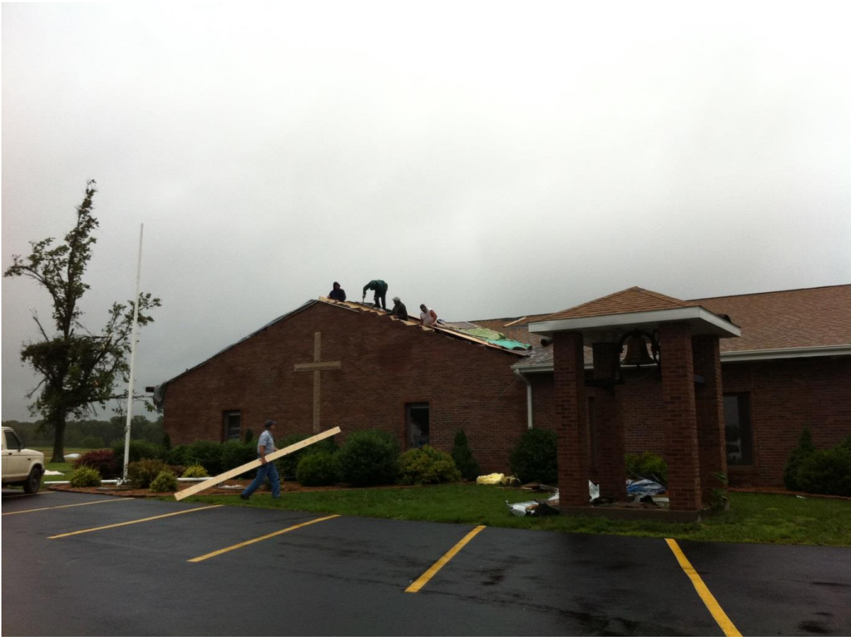
Boyd Church in repair
