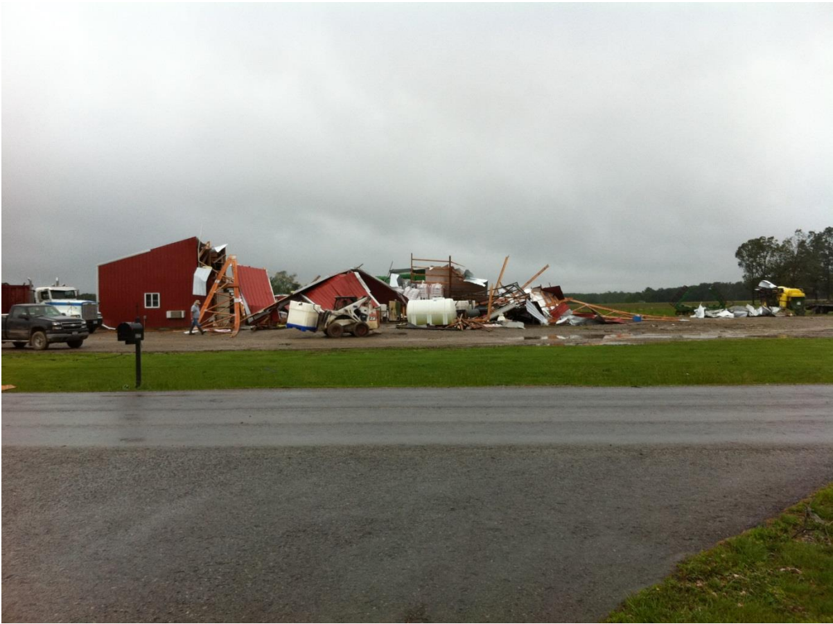
Boyd Sawmill demolished
