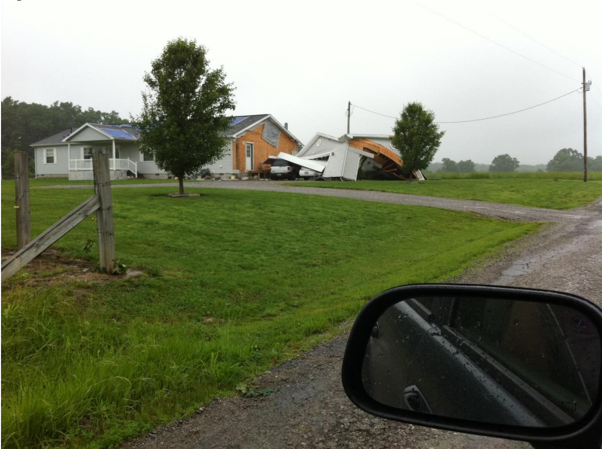
Home damaged north of Dix
