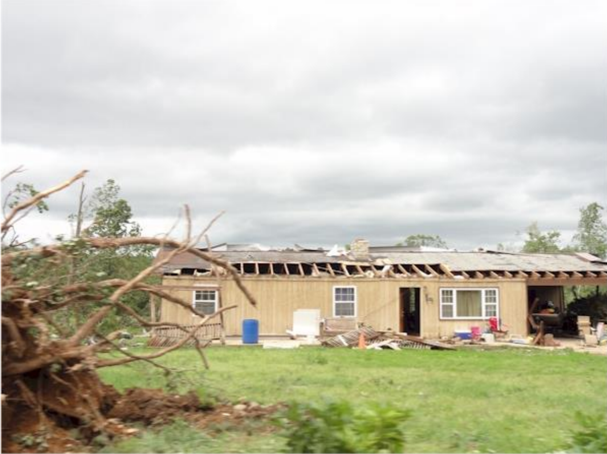
Damage to home east of Ellsinore
