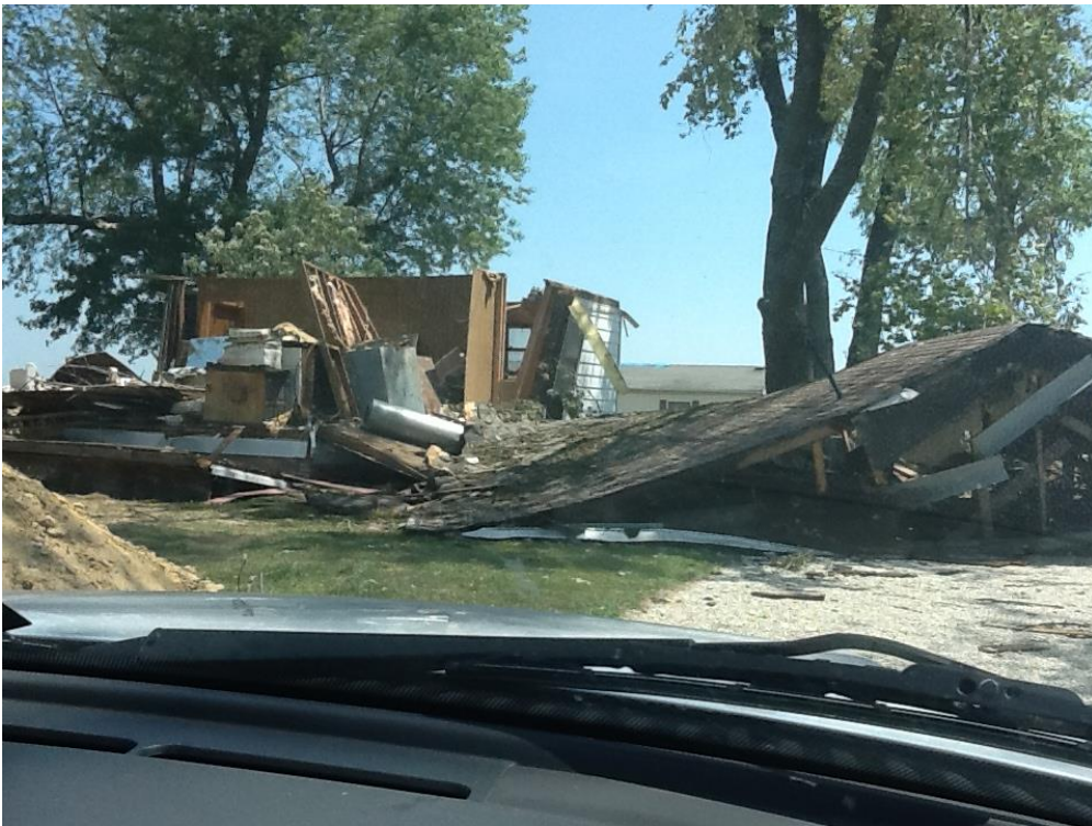
Home destroyed in Sommerville
