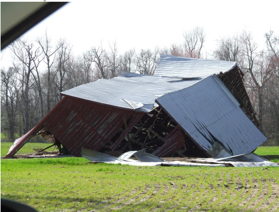
One of many barns destroyed in the path of the tornado.
