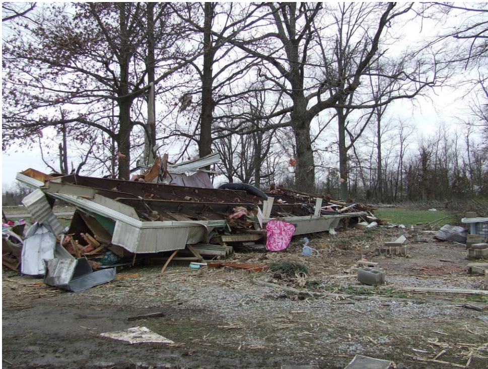
Mobile home destroyed on Odgen Landing Rd (northern McCracken County KY)
