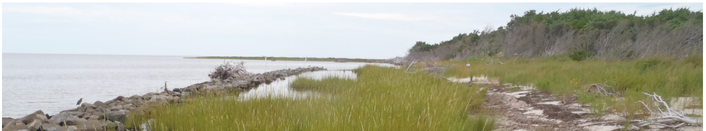
Hatteras, NC. The Durant's Point living shoreline project protects the shoreline from storm surge while providing habitat for many species. Since its construction, the project has weathered hurricanes, a summer of drought, and tropical storms. Photo: N.C. Coastal Federation
