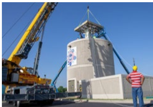
ATD Installation in Norman
