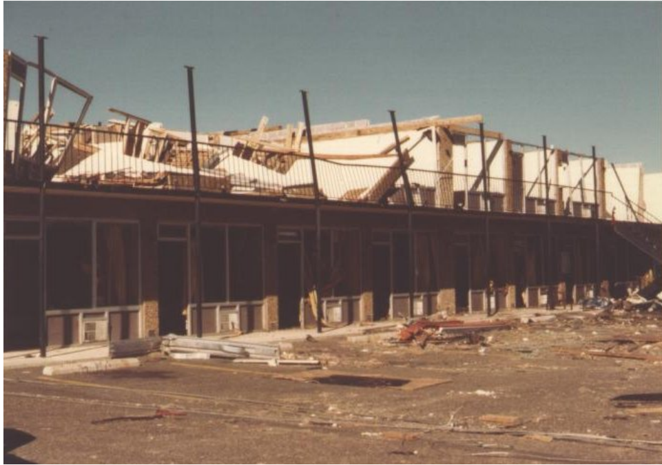
MAM: DOD 5: Collapse of top story walls
