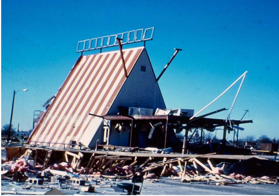
SRB: DOD 5: Canopies and covered walkways destroyed
