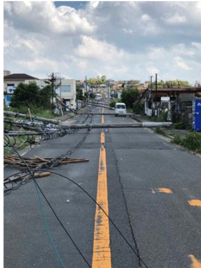
Utility poles overthrown by Typhoon Jebi (1821) (Sennan City, Osaka Prefecture)
