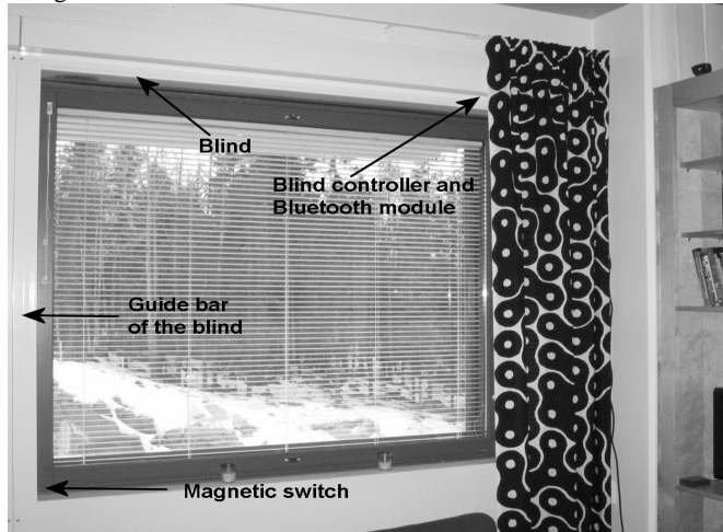
Figure 7: The components of the controllable blinder.
