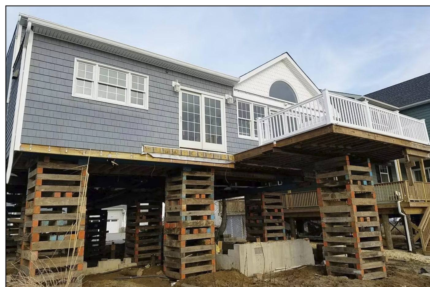
Raise building foundation to reduce flood risk.
