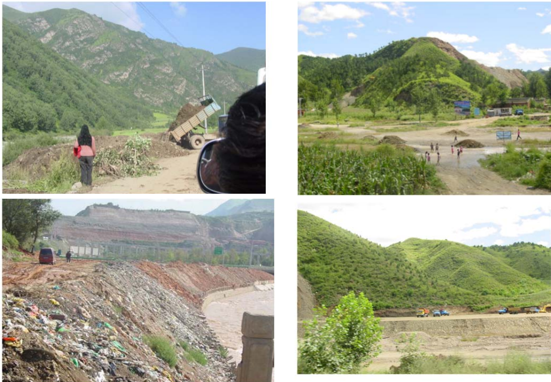
Fig. 8 Large construction projects such as roads, dams, tunnels, bridges, etc. can change river flow and water quality for a number of years. This may not be known or accountable by the modeller or the model
