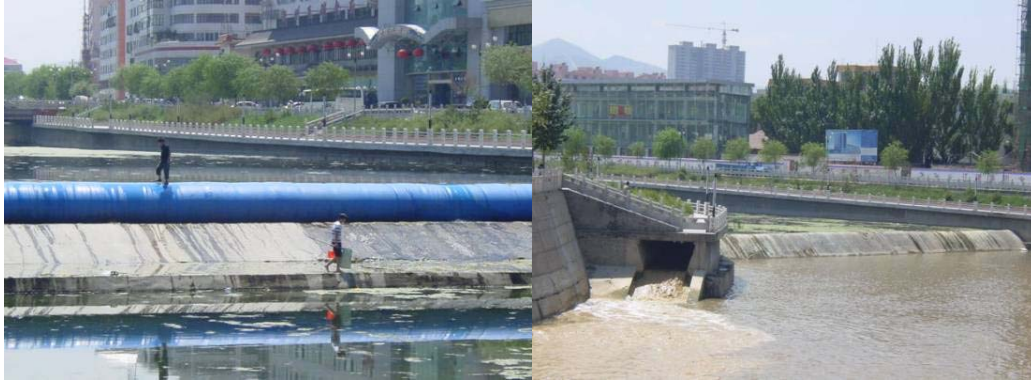
Fig. 7. Water control and water diversions may change the flow in ways that are unknown to the modeller and, hence, can not be accounted for in the model.
