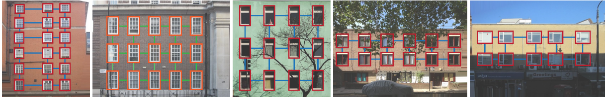
Figure 4: Extracted repetition grid in (rectified) facade images under varying regularity, occlusion, and difficult illumination conditions. In each example, the user prescribed one template rectangle W_s (top-left windows in each example). Subsequently, blind/shutter positions (not shown here) are extracted as explained in Section 4.2.
