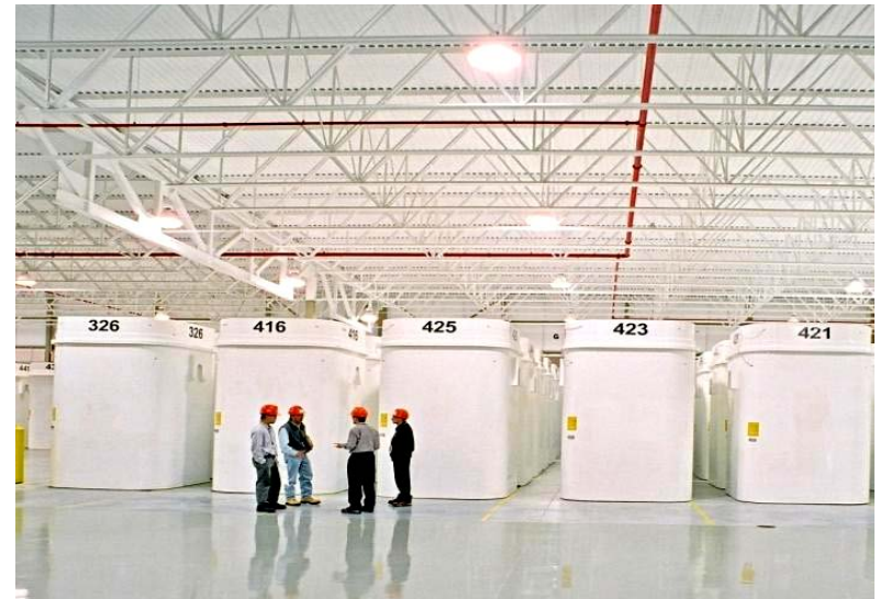
Used Fuel Dry Storage at OPG Western Waste Management Facility (Ontario)
