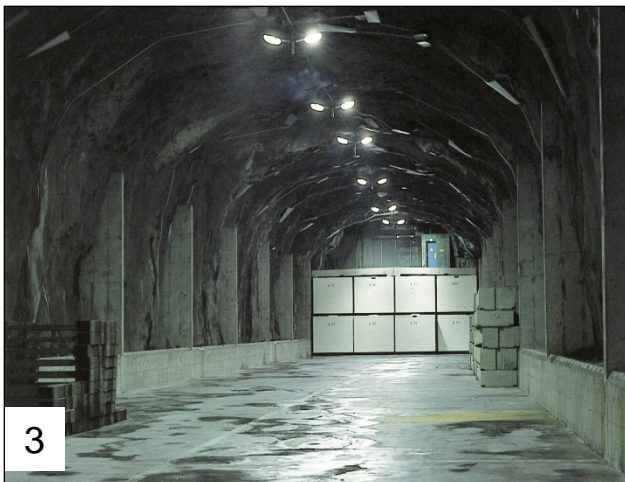
3) Sweden – SFR: near surface repository L&ILW - may ask to expand for decommissioning waste
