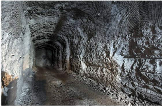
Drill and blast
